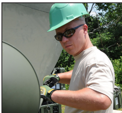
Tech. Sgt. Thomas Nancarvis, 193rd Communications Squadron, places a support rod on a satellite dish during Joint Lightning 2011 at Fort Indiantown Gap. Joint Lightning is a two week exercise that brings communications squadrons together to foster standardized operations in a combat environment. (Photo by Tech. Sgt. Matt Schwartz)
