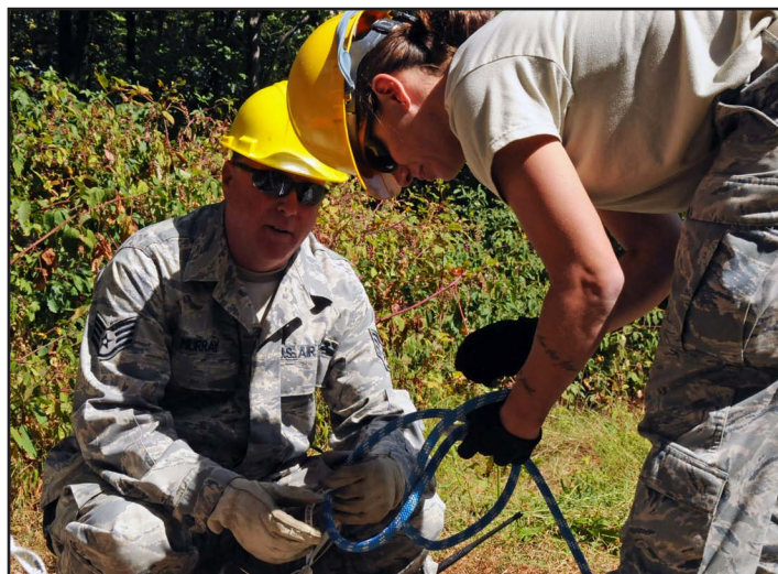
Staff Sgt. Charles Murray and Airman 1st Class Christian Dolbin, both 211th Engineering Installation Squadron, cable and antenna installers, work to secure a line to the VHF antenna so that it can be transported up the tower where four Airmen wait to attached it to the mast they installed. The installation of this antenna allowed the Airmen to get valuable on the job training to ensure they'll be mission ready. (Photo by Senior Airman Claire Behney)
